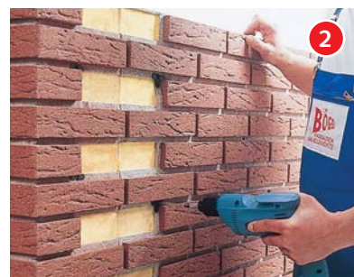
After aligning the house corner, attachment is carried out using 4 – 6 system clinker frame dowels. Attaching the panels takes place using approx. 8 bolts and through dowels in the moulded attachment sleeves designed for this purpose, which allow for the constant anchoring of the elements without placing any pressure on the thermal insulation material. Due to the stability of the complete system, screw coupling can be carried out anywhere on the joints.
