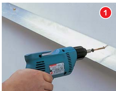
Attaching the aluminium finishing strip
