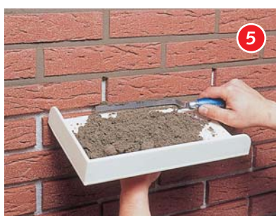
Final pointing with mortar is carried out by hand.
