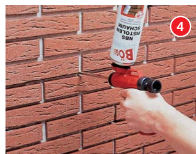
The prefabricated foam chamber ensures a uniform area coverage, free of thermal stress, through even distribution of the PU foam over all connection surfaces, transitions and irregularities on the panel longitudinal and face sides.
